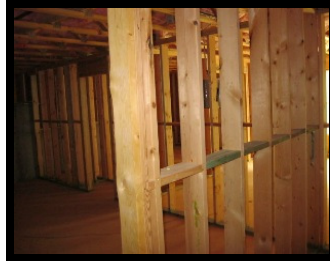
Wall Framing Structure
